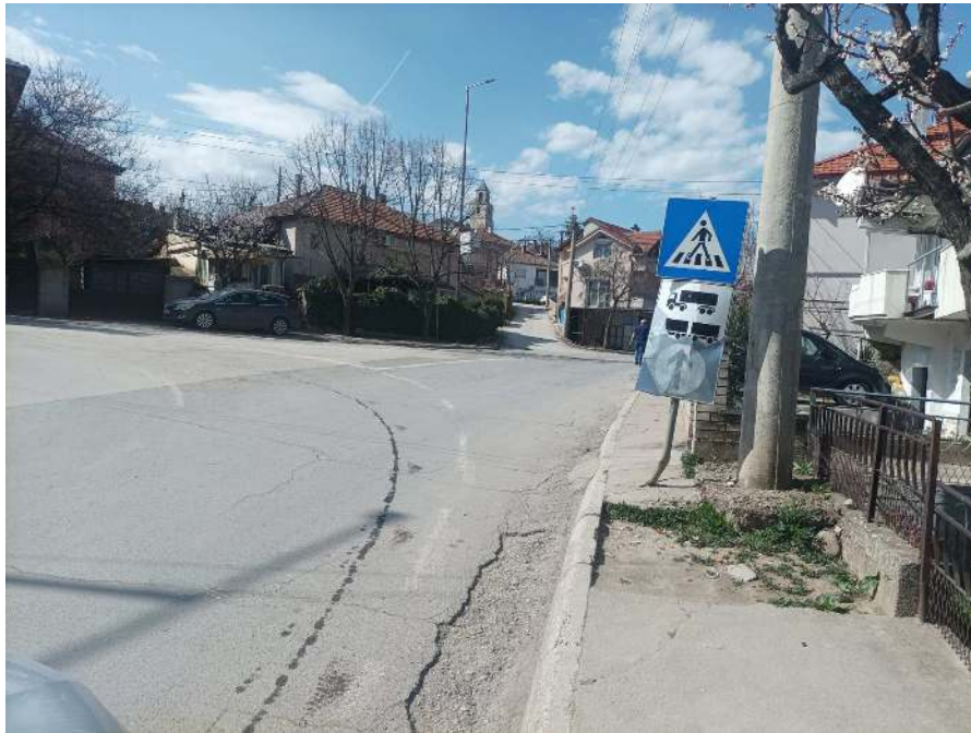
Fig.10 – End of the Part of Filip II Steet-Roundabout- km 0+1,142.30
